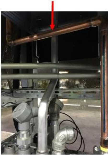
Figure 8: Maintain downward slope of newly fabricated 1" Vapor Piping.
