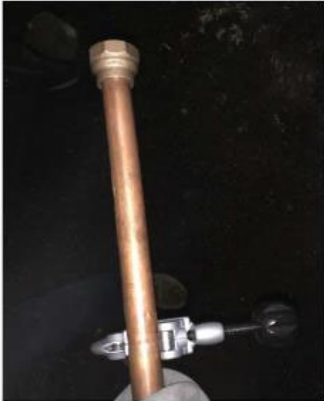
Figure 6: Cut the compression fitting from existing Vapor Piping and sweat onto new 1" copper Vapor Piping.
