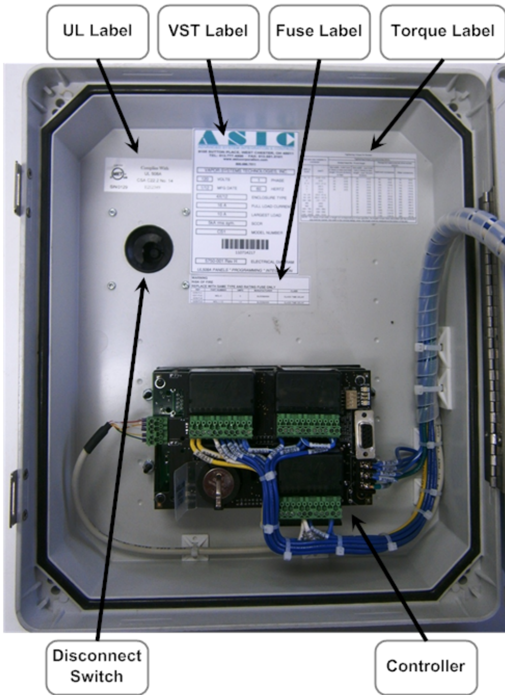
Figure 8: VST Control Panel Inside Front Cover
