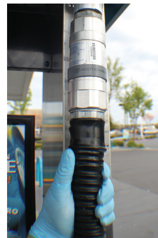
Figure 9: Verify Connection Integrity
