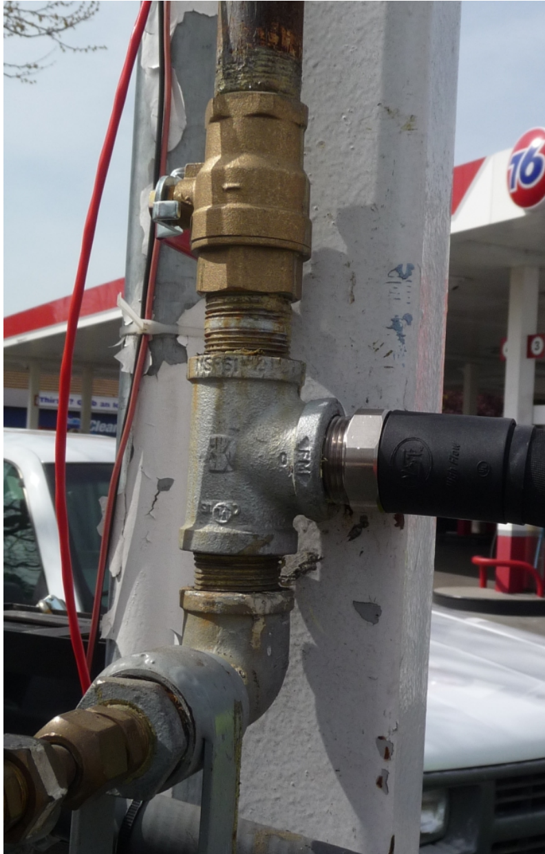
Figure 6: Test Hose on 1" Test Port
