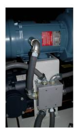
Figure 23: Blower electrical connection conduit
