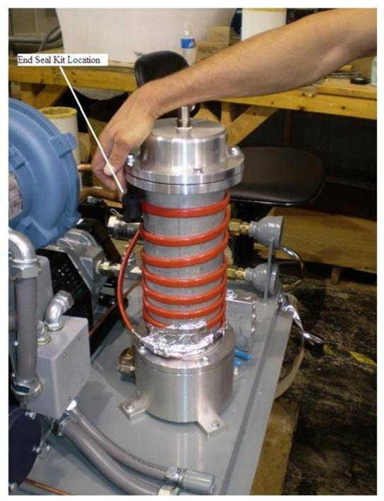
Figure 47: End seal kit location and heat trace cable installation
