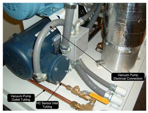
Figure 27: Vacuum pump electrical connection / vacuum pump outlet tubing / HC sensor inlet tubing
