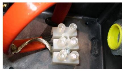
Figure 37: Termination block inside the electrical junction box
