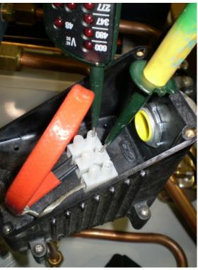
Figure 16: Heat Trace Circuit Test
