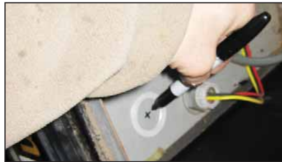
Figure 5: Mark Drilling Location
