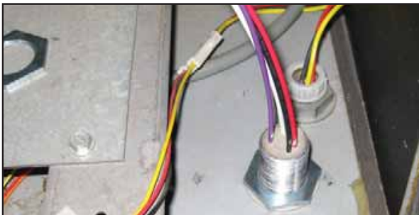
Figure 7: Potted Nipple Assembly Attached
