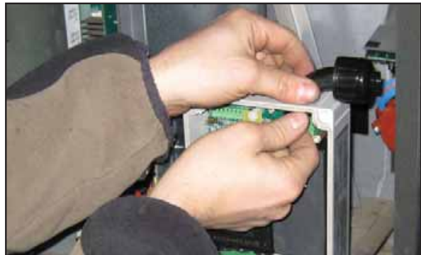
Figure 9: Attach 90-degree Fitting
