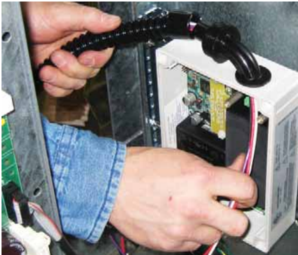
Figure 15: Attach Flexible Conduit to 90-Degree Fitting
