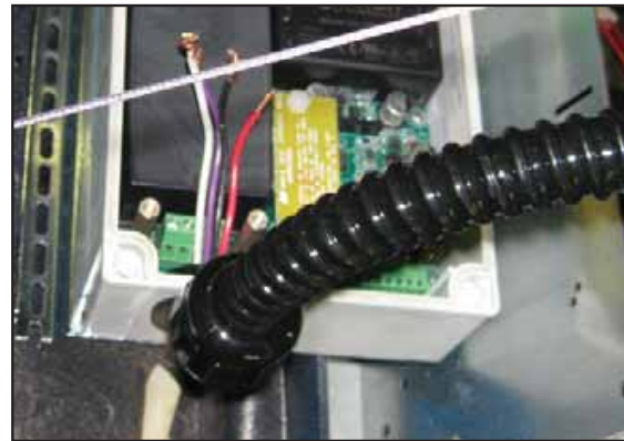
Figure 12: 90-Degree Fitting Installed
