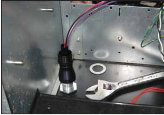
Figure 5: Straight Conduit Installed
