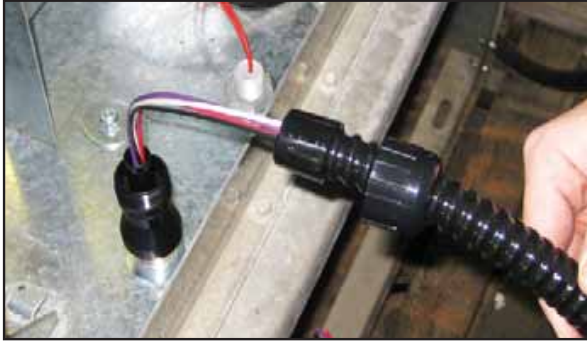
Figure 14: Attach Flexible Conduit to Potted Nipple
