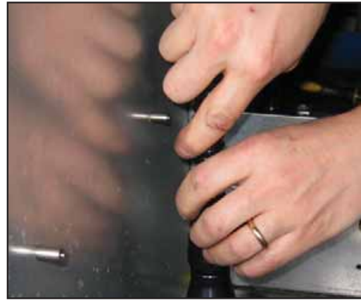
Figure 11: Flexible Conduit Installation
