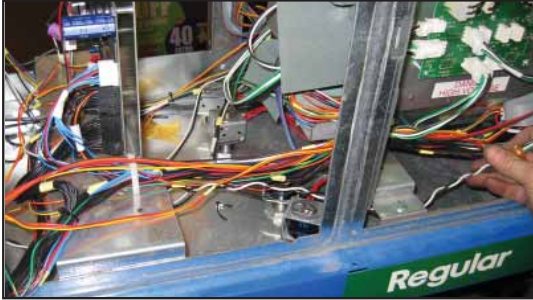
Figure 16: Power Cable Installation
