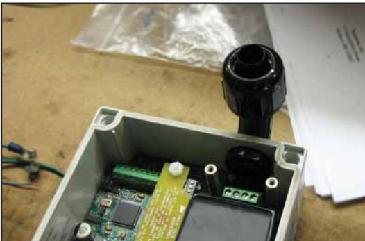
Figure 7: 90-Degree Fitting Installed
