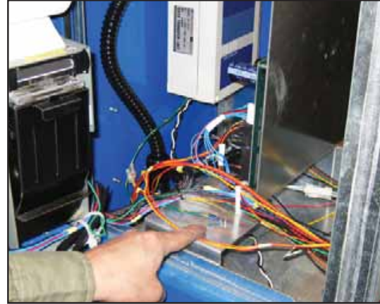
Figure 18: Ground Wire Attached
