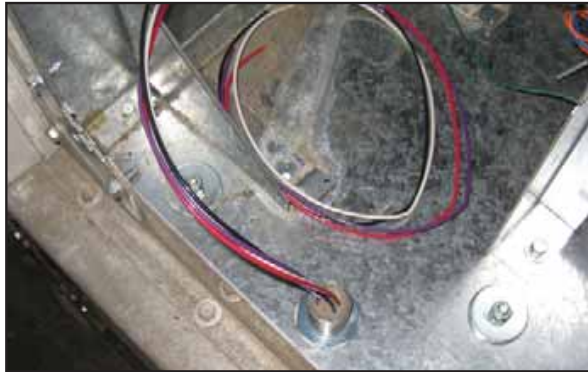
Figure 11: Install Potted Nipple
