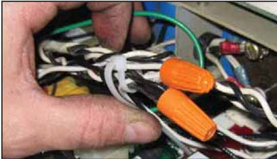
Figure 11: Wrap Wires
