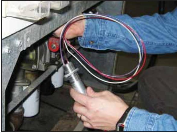
Figure 10: Push Wire to Electrical Enclosure
