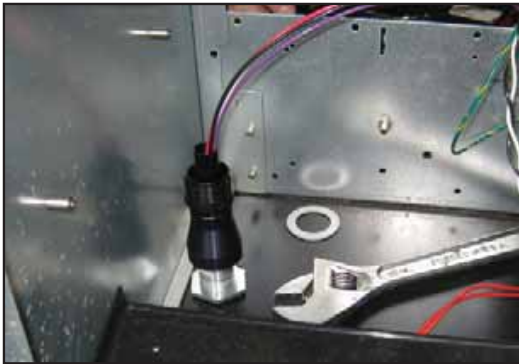
Figure 6: Straight Conduit Installed
