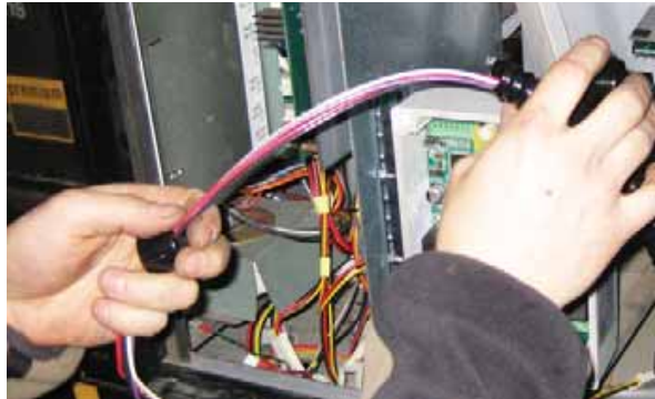
Figure 11: Attach Flexible Conduit to 90-Degree Fitting
