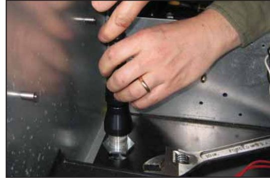
Figure 14: Attach Flexible Conduit
