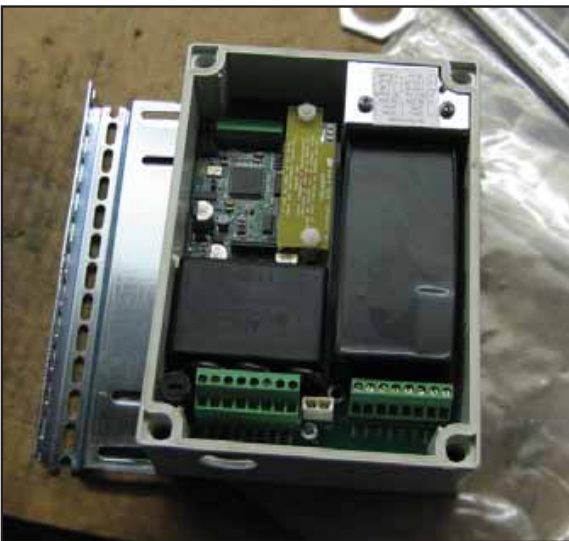
Figure 2: Mounting Bracket Installed
