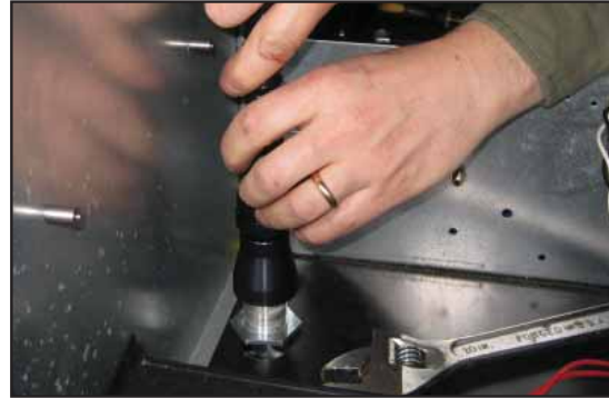
Figure 13: Attach Flexible Conduit
