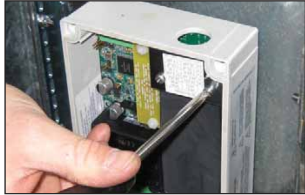
Figure 12: Remove Wiring Cover
