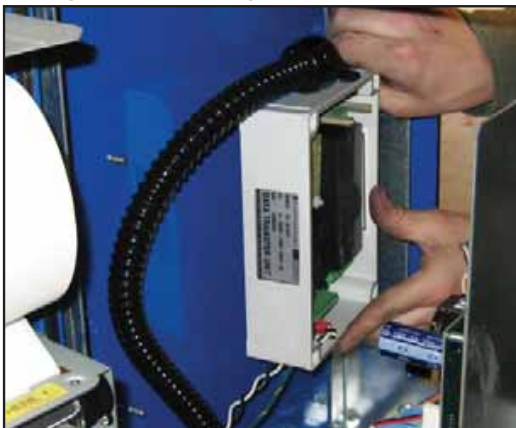
Figure 13: 90-Degree Conduit Connected
