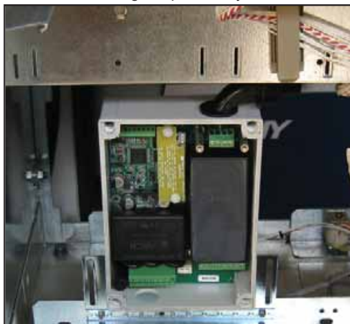
Figure 11: 90-degree Fitting Installed
