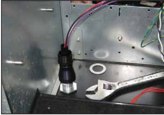
Figure 6: Straight Conduit Installed
