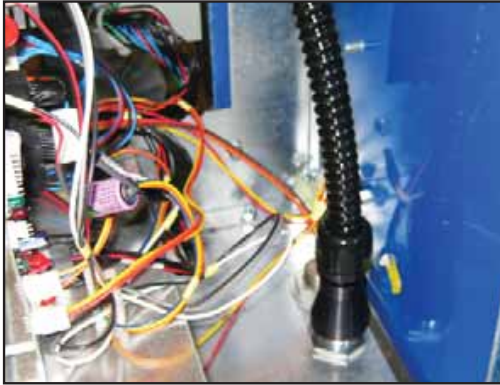
Figure 11: Flexible Conduit Connected
