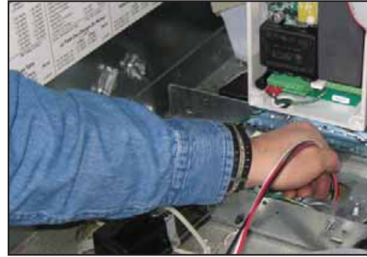
Figure 8: Pulling Wires Through Opening
