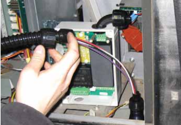
Figure 10: Attach Flexible Conduit to Potted Nipple
