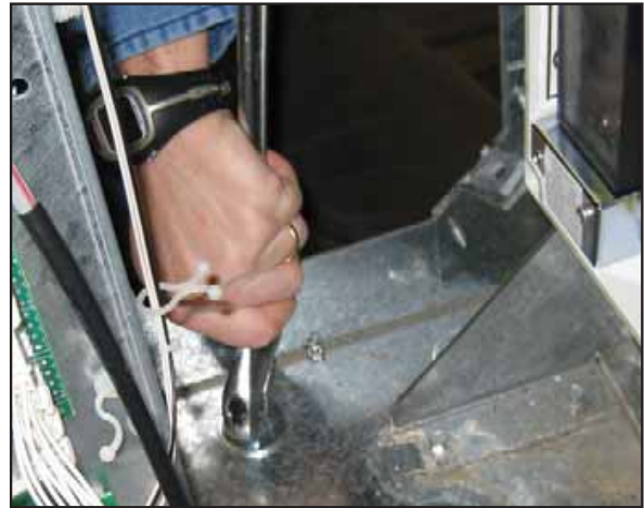
Figure 8: Remove Hole Plug
