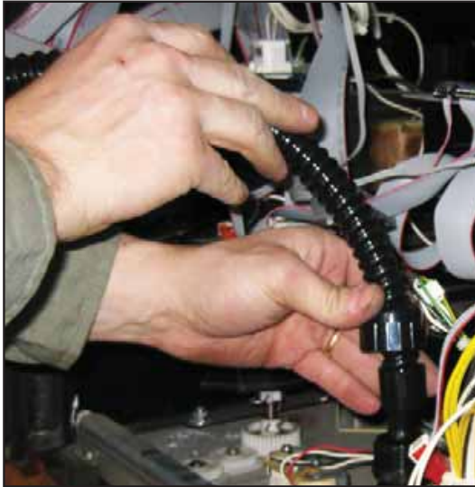
Figure 12: Attaching Flexible Conduit
