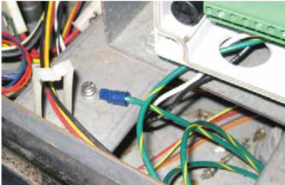
Figure 16: Attach Ground Wire
