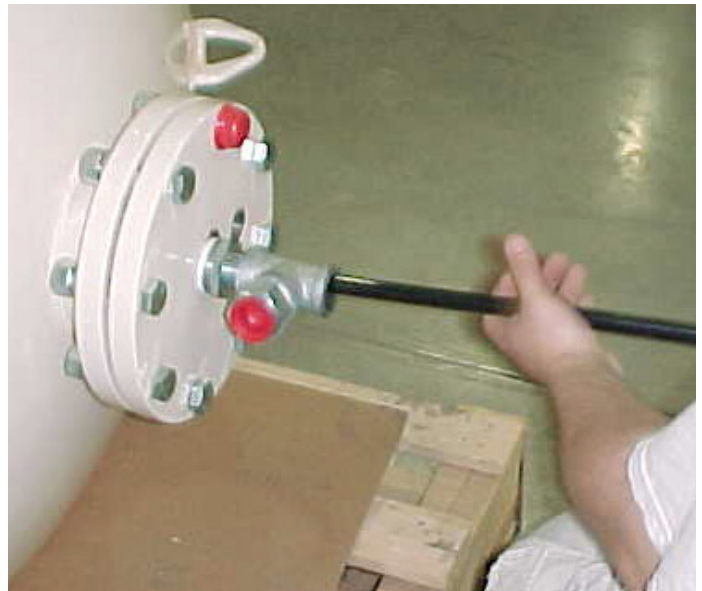
Figure 4: Install Syphon Tube
