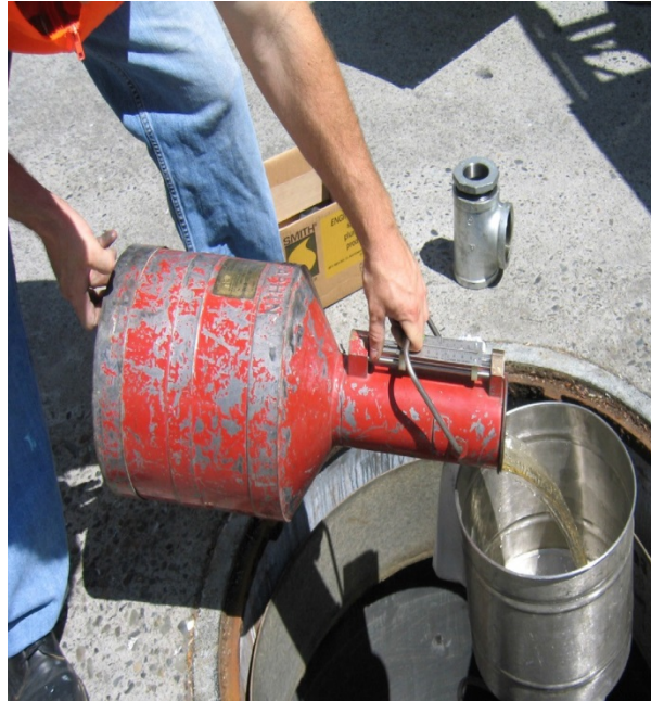
FIGURE 9-3 Adding Gasoline through Open Fuel Entry Point
