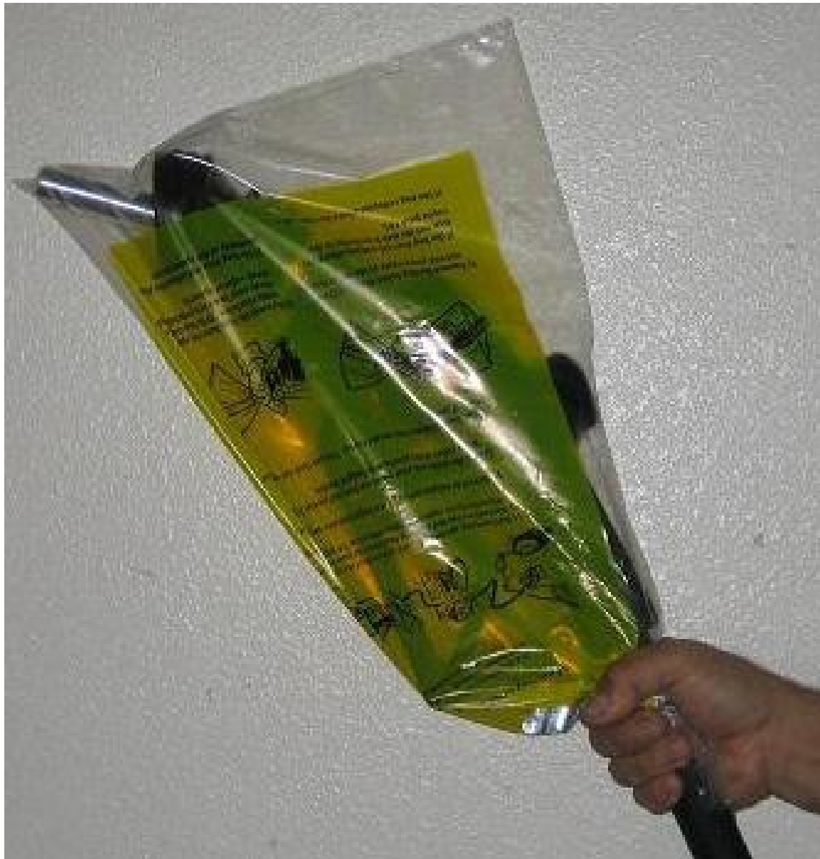
FIGURE 7-1 Typical Example of Bagging a Nozzle
